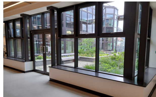
Windows on the ground floor of Catkin Centre
